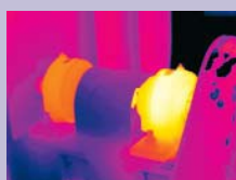
Overheating bearing cap
