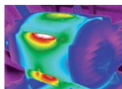
Abnormal/uneven heating on motor
